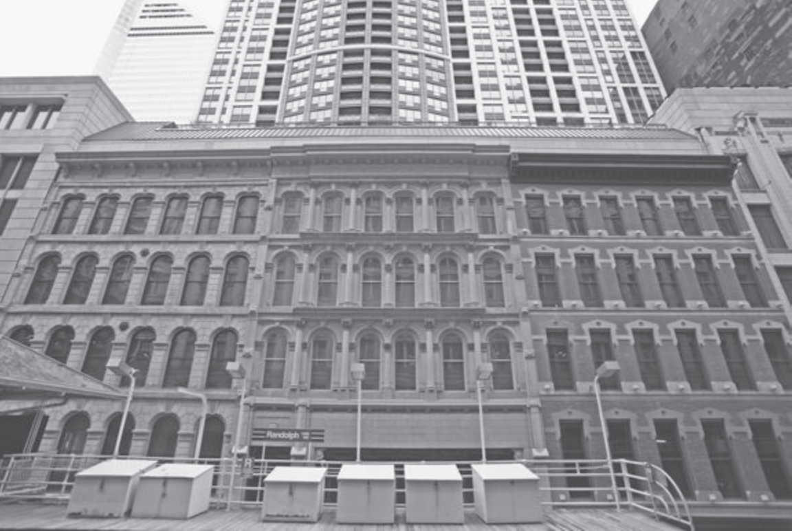
HISTORIC FACADES ON CHICAGO'S WABASH AVENUE Saving a streetscape, but wreaking havoc on architectural integrity.
