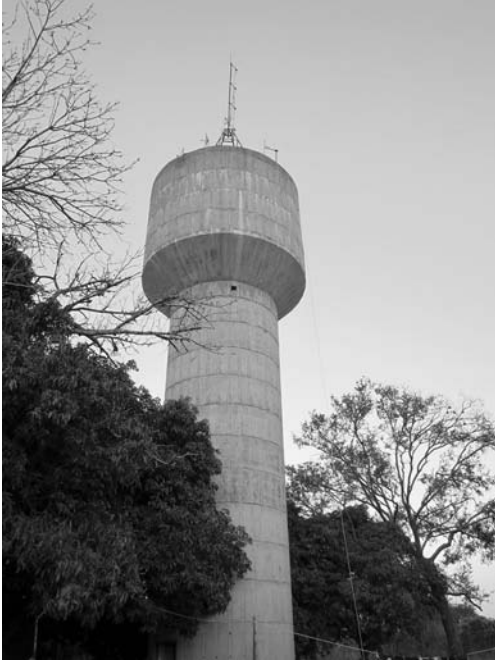
Figure 5.6. Macha's water tower hosts several antennas and was one of the sites of our team's VillageCell experiment. Photo by author.
