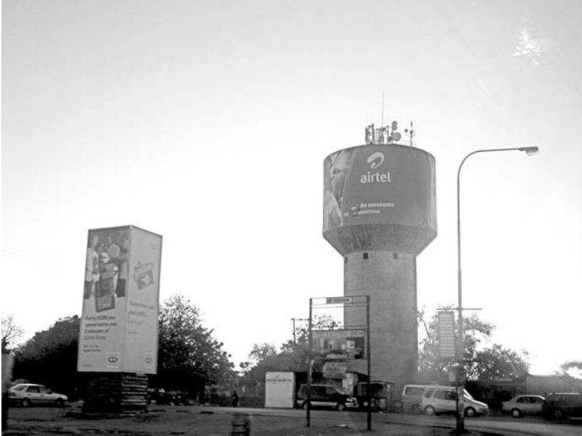
Figure I.2. In Lusaka, Zambia, mobile phone providers lease space on water towers to send signals and advertise their services.
