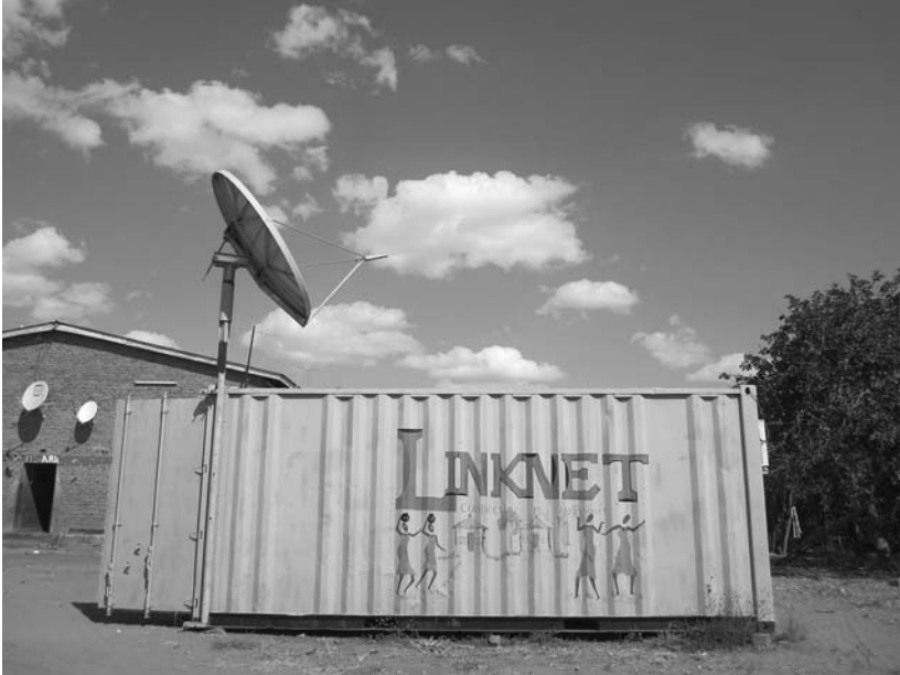
Figure 5.2. Machans could access the Internet from 2011 to 2012 from several LinkNet VSAT terminals built out of repurposed cargo containers. Photo by author.
