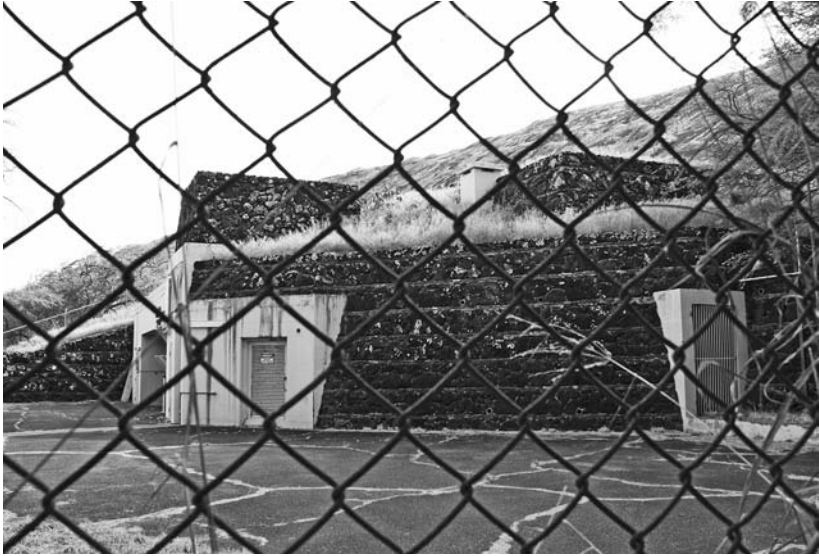
Figure I.3. At Hanauma Bay, Hawai'i, a Cold War–era undersea cable station was buried underground in order to protect it from attack.
