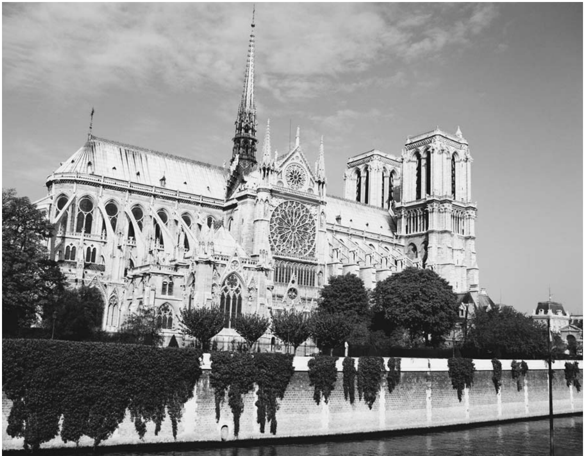
The Cathedral of Notre-Dame located in Paris, France, is an example of a Gothic cathedral. Note the flying buttresses (left) supporting the cathedral's ceiling and walls. ( Getty Images )
