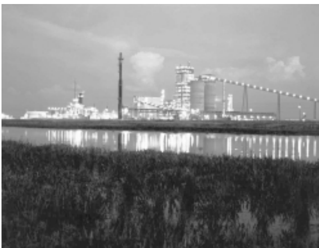
Figure 1.14. Tampa Electric's Polk IGCC Power Station Unit 1. Photo courtesy of Mr. Mark J. Hornick of Tampa Electric.
