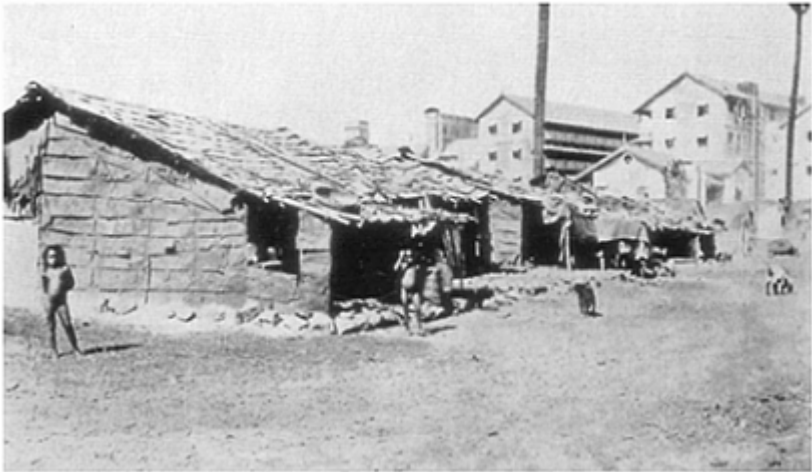
Temporary houses for workers in Bombay. In the foreground are sheds made from flattened kerosene tins, in the background chawls built by the colonial authorities. (Source: Burnett-Hurst, 1925)
