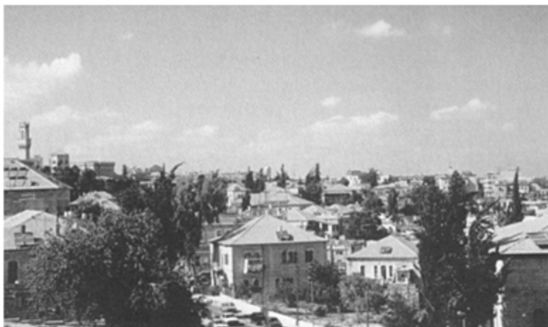
Low-density garden suburb housing in Tel Aviv. Patrick Geddes planned several such layouts in the 1920s as consultant to the Zionist Organization. (Source: The author, photo taken in 1992)
