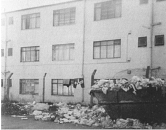
Exterior of African hostels in Guguletu (Cape Town). Designed on the barrack principle for single-workers, they now accommodate families in grossly overcrowded and insanitary conditions. (Source: The author, photo taken in 1995)
