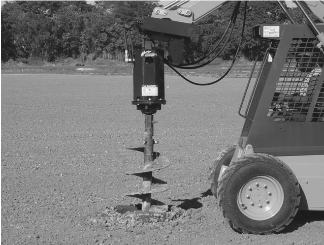
FIGURE 7.5 Auguring a cylindrical hole into the soil or limestone bedrock to depth so that the top of the lysimeter is below crop roots.
