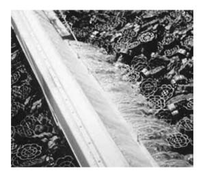
**FIGURE 3-17.** Photo of a rotating distributor of trickling filter with random plastic media. (Courtesy of Jaeger Environmental, www.jaegerenvironmental.com/)
