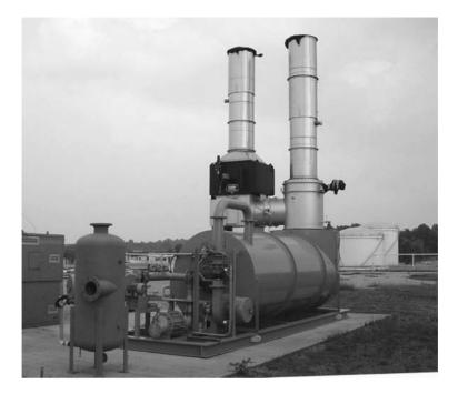
**FIGURE 6-10.** Large gas-fired thermal/catalytic oxidizer. (Photograph provided by Intellishare Environmental, Inc.)
