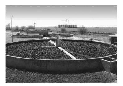
**FIGURE 3-16.** Photo of a trickling filter with random plastic media. (Courtesy of Jaeger Environmental, www.jaegerenvironmental.com/)
