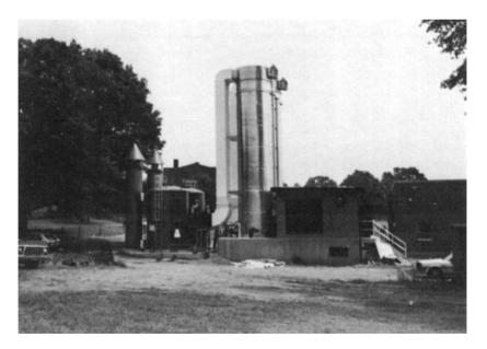
FIGURE 2-18. Packed-tower air stripper with VPGAC.
