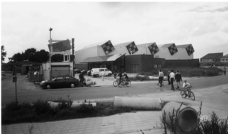
Figure 7.10 Sports centre with PVs on the roof and on the bike shelter
