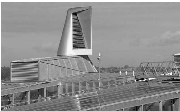
Figure 14.16 Nottingham University wind cowls with photovoltaic atrium roofs in foreground
