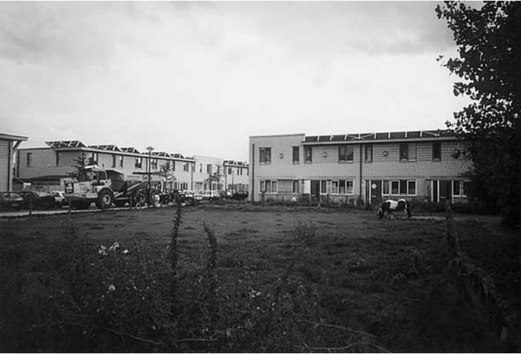
Figure 7.6 Free-standing PV modules on roofs, one dumper-truck and a pony
