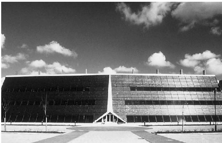
Figure 1.2 Solar Office, Doxford (Sunderland) (see Chapter 10)
