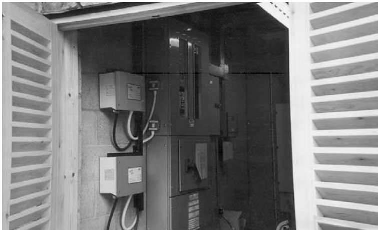
Figure 5.3 Alternative inverter arrangements
