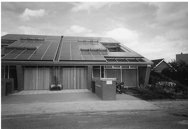
Figure 7.5 PV modules on the roof of the Energy Balance Home (and some opening windows)
