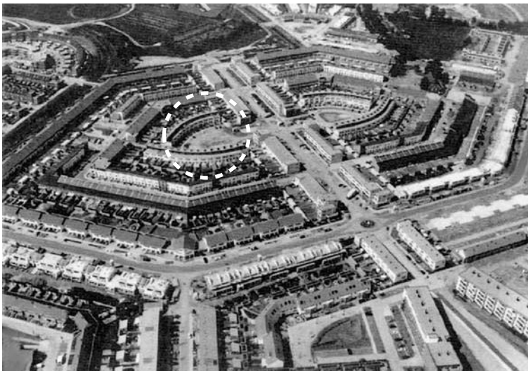
7.1(b) Area of PV roofs
