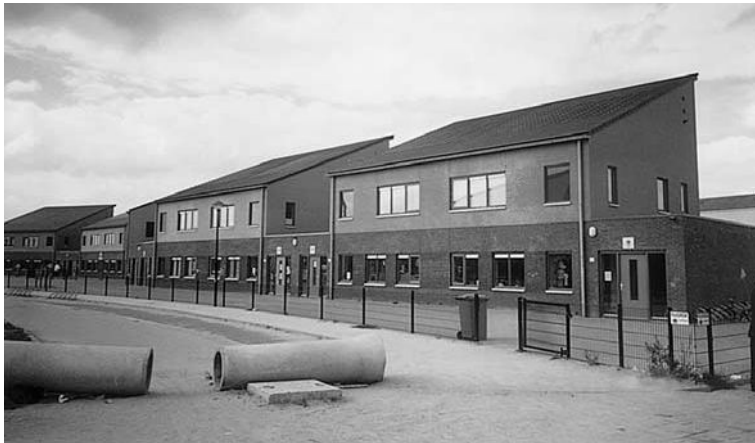
Figure 7.9 PV roofs on a building currently used as a school
