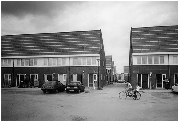
Figure 7.4 PV modules on roof
