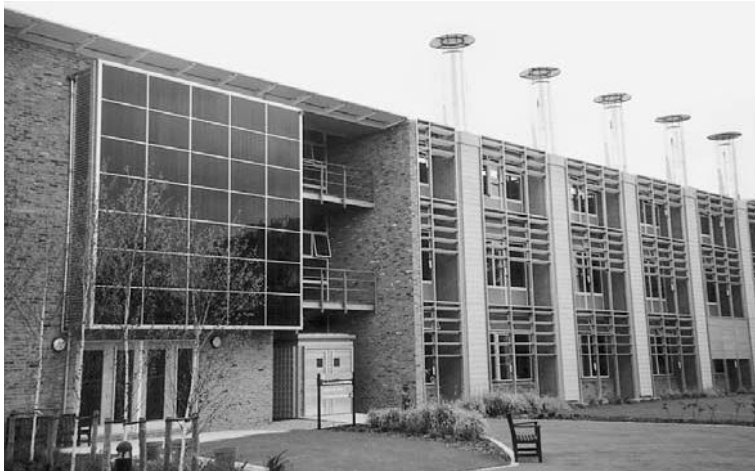
Figure 5.2 PV installation at the BRE Environmental Building
