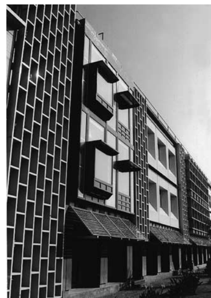
Figure 14.12 Conphoebus low-energy office building with two-storey test facade
