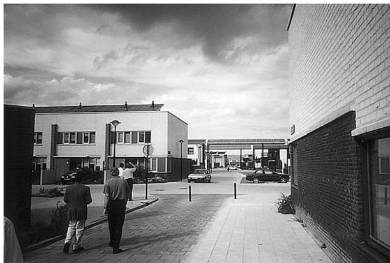
Figure 7.2 PV modules on roofs (on homes to the left)
