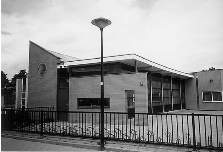
Figure 7.3 PV modules on roof of a school
