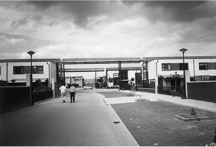
Figure 7.8 Steel bridging structures with PV arrays
