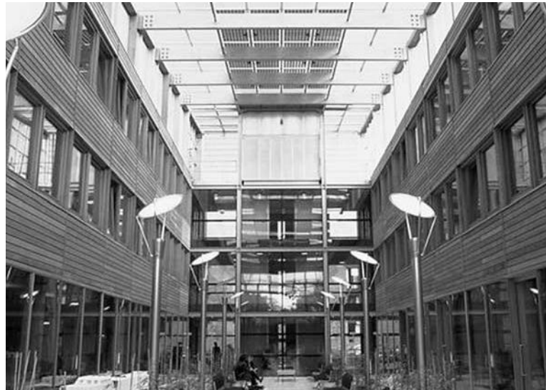
Figure 14.18 PV mounted on the atrium roof at the University of Nottingham (Architect: Michael Hopkins and Partners)
