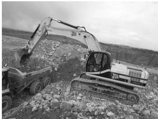
(c) A JCB UK Ltd. tracked excavator ( www.jcb.com )
