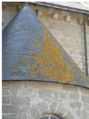
FIG. 15.12. – Colonization of a roof by orange lichens.
