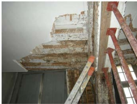
FIG. 15.14. – Drilling to check the health status of the woods.
