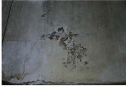
FIG. 15.6. – Ryzhomorphs of Coniophora puteana emerging from a wall.
