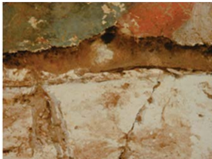
FIG. 15.5. – Dry rot filaments on a wall painting.
