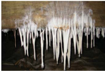
FIG. 15.7. – Development of Poria placenta on a beam.
