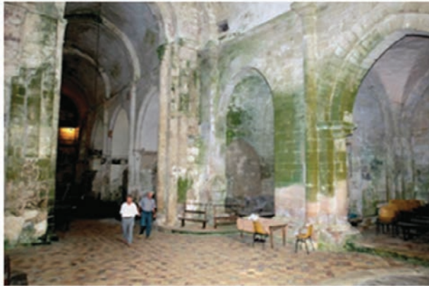
FIG. 15.11. – Interior of the Salles Lavauguyon church (France), the walls and pillars of which are highly colonised by algae.
