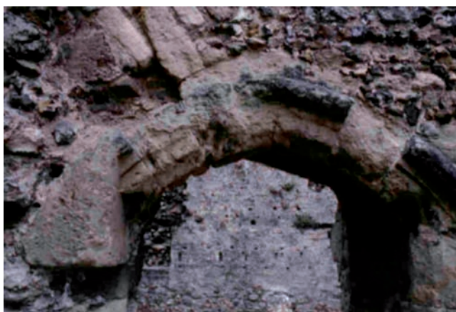
Figure 7 Stone decay and crusts on decorative arches at Portchester Castle associated with high counts of microorganisms
