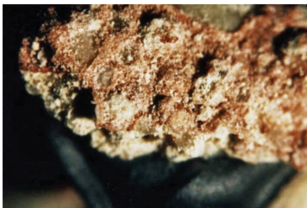
Figure 4 Flaking of paintlayer, sample from Gnoiden, Germany
