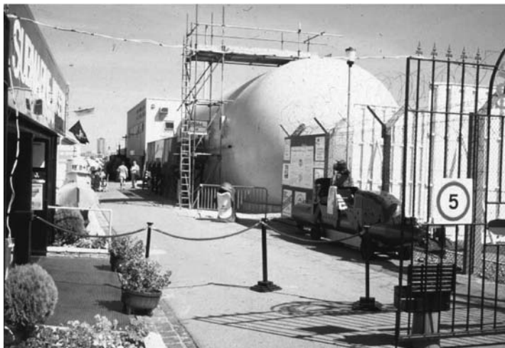
Figure 9 The complete cell formed around Holland 1 for aqueous washing of the chloride ions from the submarine
