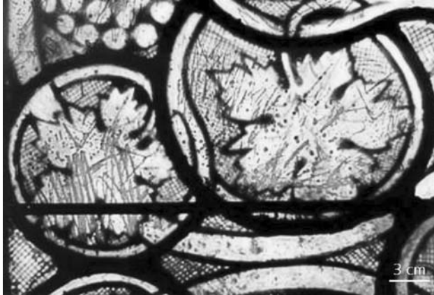
Figure 11 Scratches on a stained glass from Cologne Cathedral, resulting from a previous cleaning process
