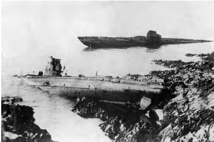
UB86 and UB112 beached at Falmouth in early 1921 after being damaged in the explosive trials. (C B 1622)
