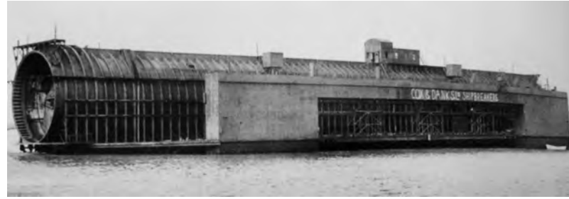
The first of the 'pressure' or 'tubular' docks to be built by the German navy (Brückenbau Flender 21) to pressure-test submarine hulls. Unlike a second example, which never reached the UK, this one was acquired by the shipbreakers Cox & Danks and, after the removal of the pressure-cylinder, reconfigured as a salvage-platform. (AD collection)
