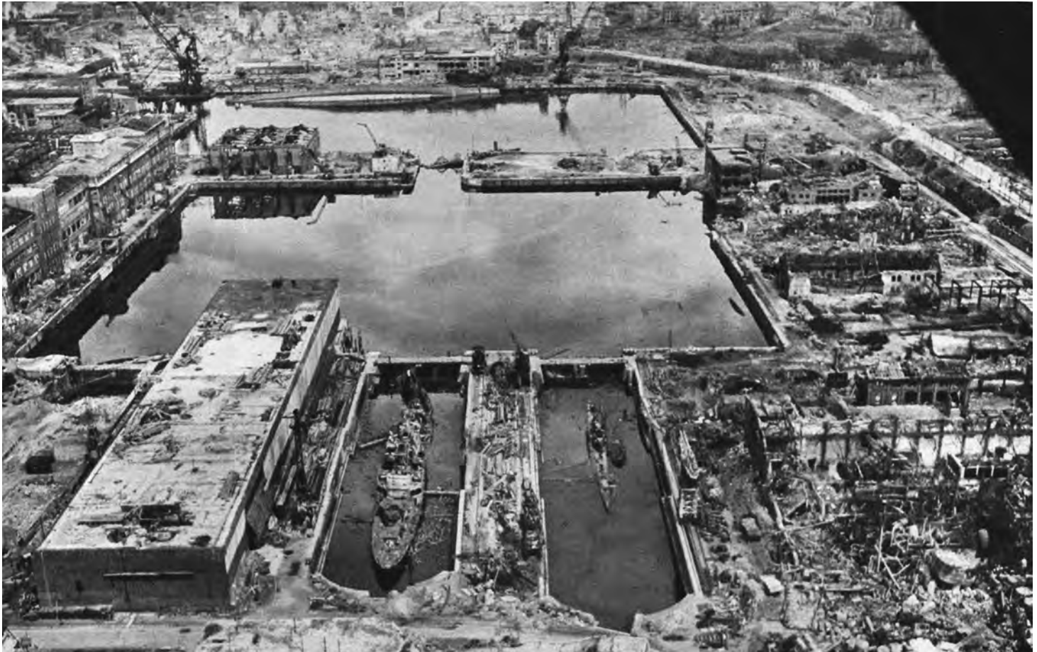
The Deutsche Werke, Kiel, in May 1945: view from the west, with, from the left: the partly filled-in Dock IV; the 'Konrad' submarine construction and repair bunker, built over the former Dock III; the wreck of Brummer in Dock II; and U1166 in the adjacent Dock I. The capsized wreck of Scheer is visible in the background, in the Innerhafen. The partly-scraped remains of Brummer and Scheer were subsequently buried when the docks were filled in, although that of the former was exposed again when the new Howaldtswerke yard was being built directly to the west in the early 1960s; during this time the 'Konrad' bunker was finally demolished. (AD collection)
