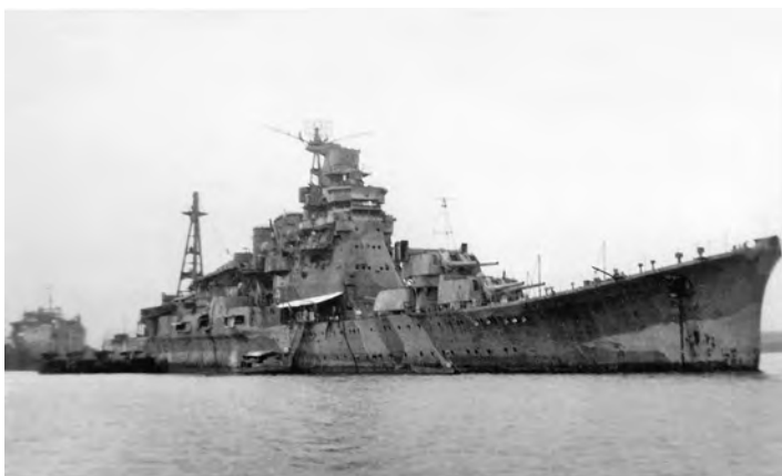
Takao at Singapore in 1945 after her surrender to the British. During the Battle of Leyte Gulf, on 23 October 1944, she had been hit by two torpedoes from USS/M Darter , which had blown off her stern (see p 199) and flooded three boiler rooms; she arrived at Singapore on 12 November. Since there was no possibility of getting her back to Japan for repairs, she was employed as a floating AA battery, with reduced crew and all 203mm ammunition landed; it was at this time that the ship was camouflaged. She was subsequently attacked by HMS/M XE3 on 31 July 1945, which deposited a 1-ton mine and limpet mines below her, blowing a 7 x 3m hole in her bottom, flooding a number of compartments and unseating a number of turrets and rangefinders. (AD collection)
