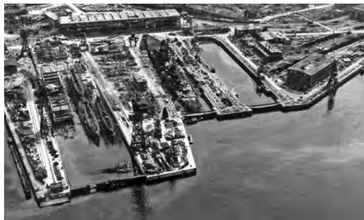
The Deutsche Werke, Kiel, in May 1945: view from the north, with the empty Dock VI on the right, Hipper in Dock V in the centre, and the suspended Type XIV submarine tankers U491 , U492 and U493 on the slip on the left. (AD collection)
