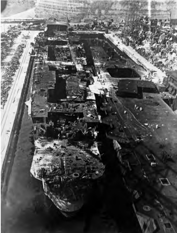
The aircraft carriers Kasagi and Ibuki being broken up at Sasebo in early 1947. Kasagi was another ship of the Unryu class, and had been suspended when 84 per cent complete on 1 April 1945, while Ibuki has been laid down as a heavy cruiser, but converted to a carrier after launching; she was suspended when 80 per cent complete on 16 March 1945. (NHHC NH 85887)
