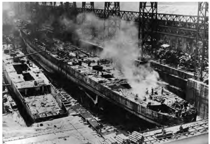
Oyodo being broken up in dry dock at Kure on 27 April 1948. (NHHC NH 111636)
