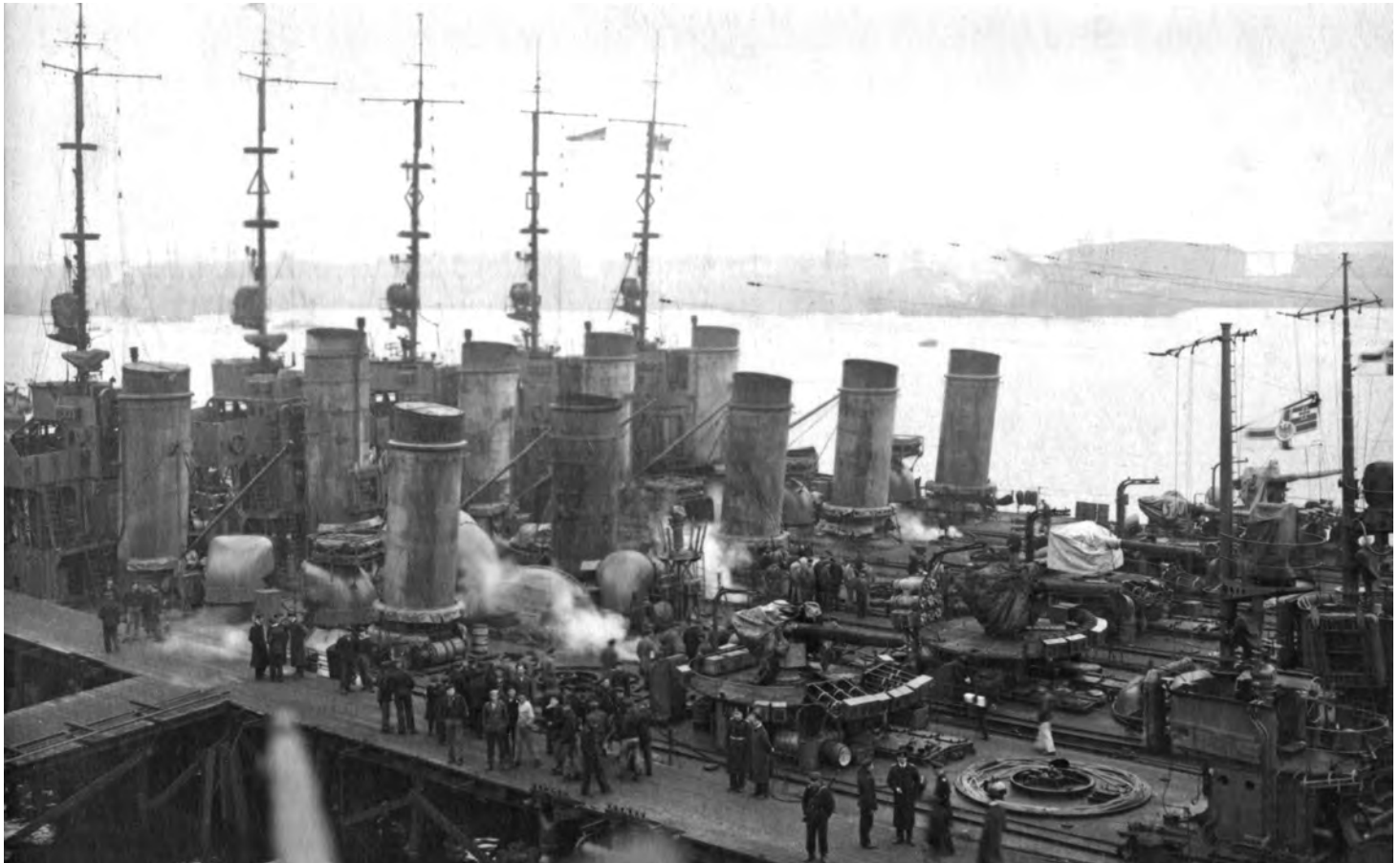
Members of Germany's active destroyer force of the immediate post-war era, the so-called Eisernen Flotille, on 24 February 1919. Second from the left is V79, the remaining ships being S133, S134, S135 and S136; note the absence of torpedo tubes, removed from all vessels to meet Armistice requirements. All still fly the old Imperial ensign, the new Reichsmarine ensign not being introduced until 1921. (AD collection)
