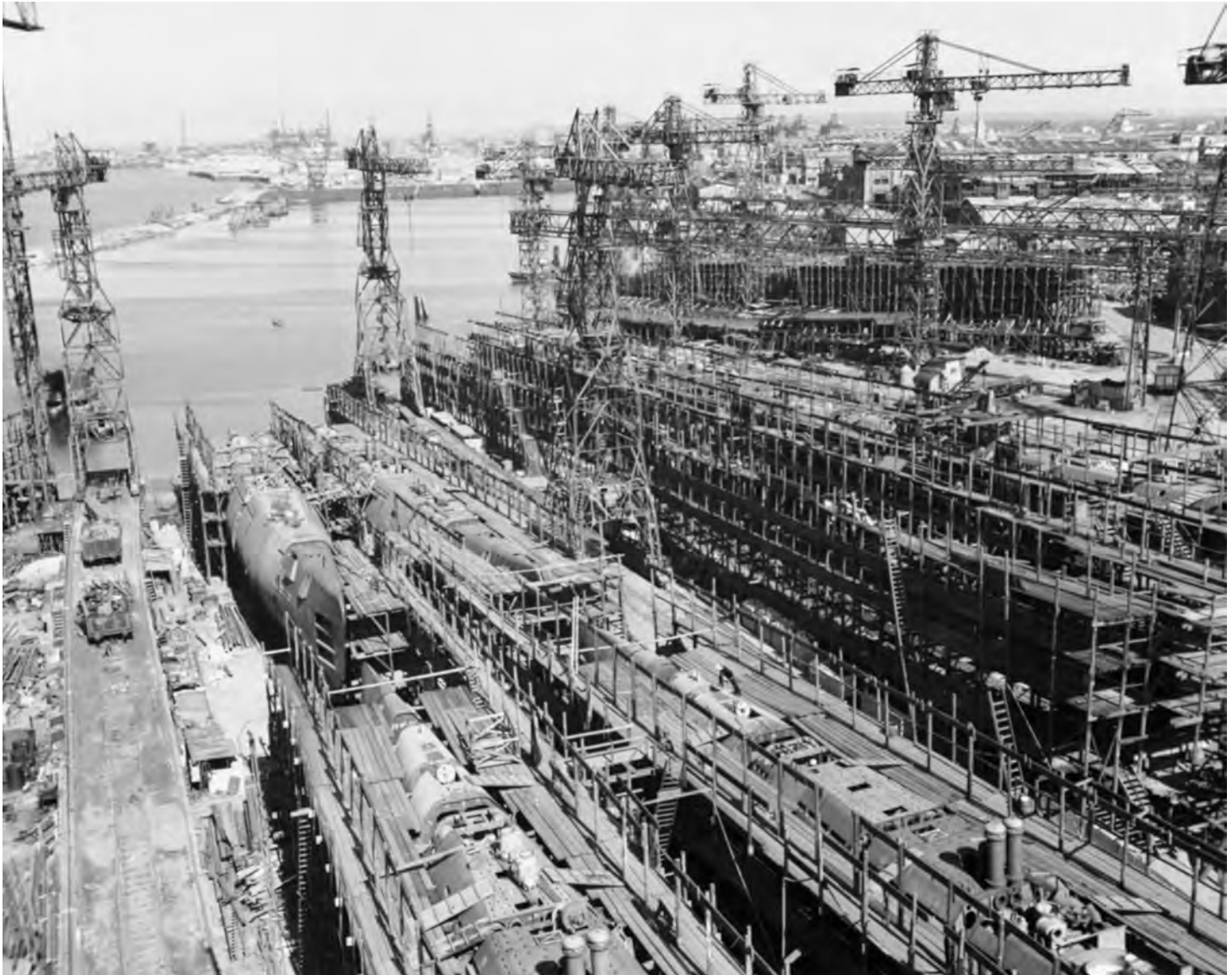
Bremen after its capture in May 1945, showing Type XXI submarines on the slips of the Deschimag yard. (NHHC 80-G-333672)
