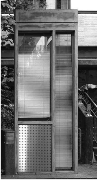
Figure 6 Modular façade element, Knaack, Bilow 2004. Glassfiber reinforced concrete with decentralized climate unit
