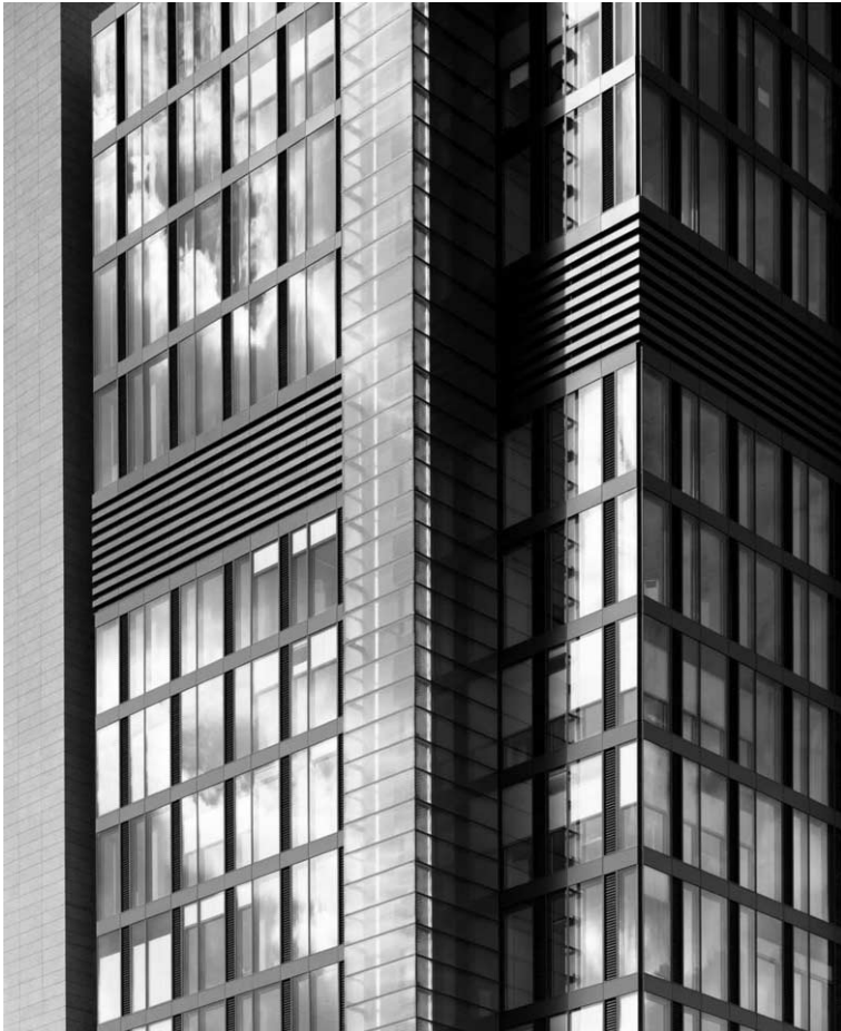
Figure 3 debitel Headquarter / Stuttgart – a combination of an boxed façade unit with a single layered façade, the so called “hybrid façade”
