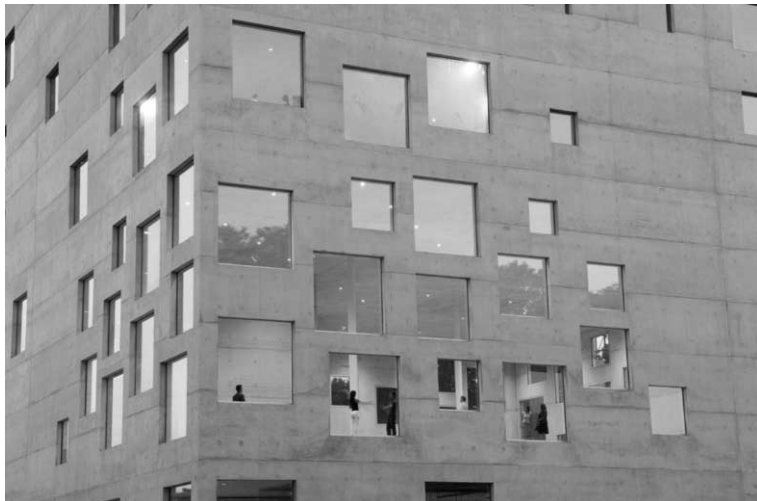
Figure 9 Building upon completion
