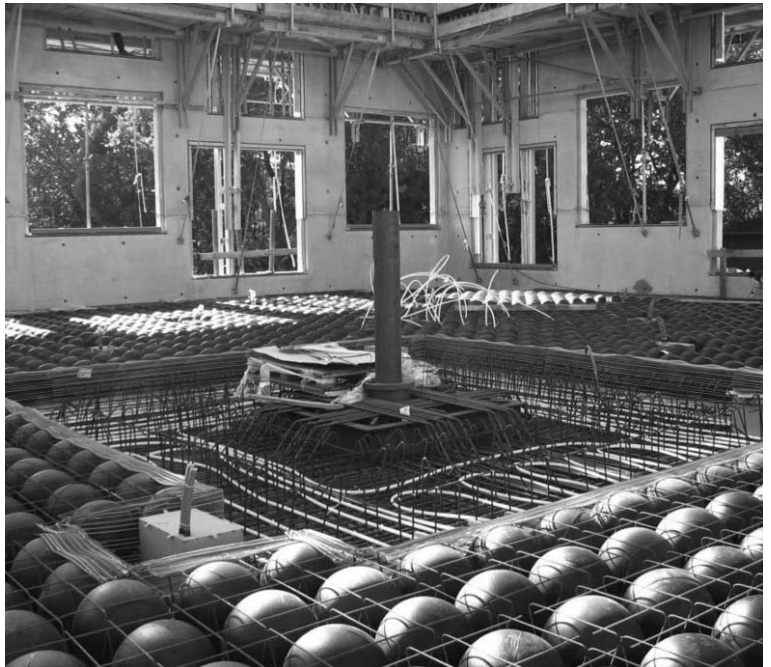
Figure 3 Lower reinforcement layer, piping for activated building components, displacement bodies, built-in light fixtures
