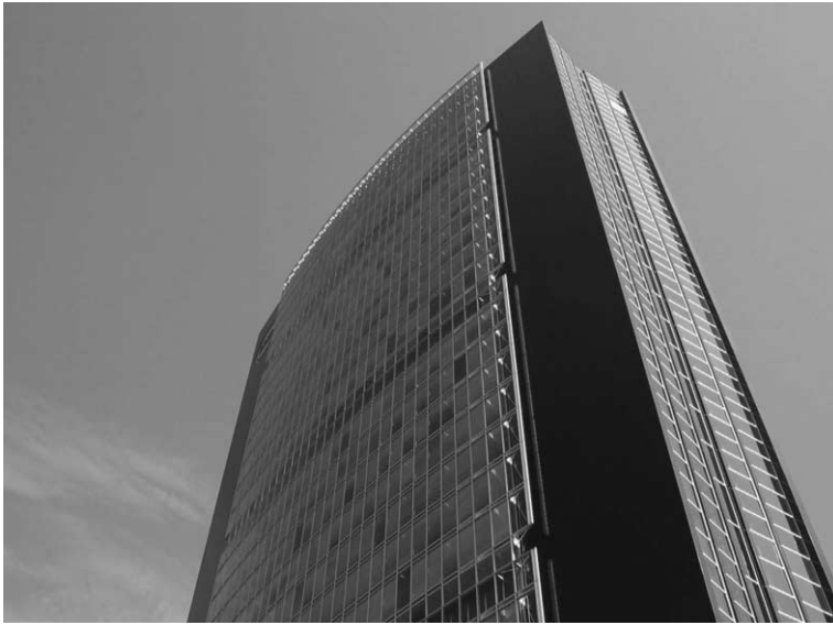
Figure 2 ARAG Tower / Düsseldorf – a combination of a story-spanning chimney in the façade cavity and boxed window units to provide individual ventilation possibility
