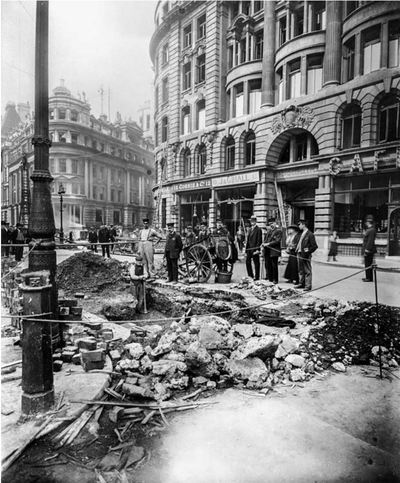
2.1 Damage to Liverpool Street in London following the Zeppelin raid on the night of September 8–9, 1915. Messrs Niles and Kaye, London, 1915. LC 32. Corporation of the City of London Collection, Imperial War Museum, London.
