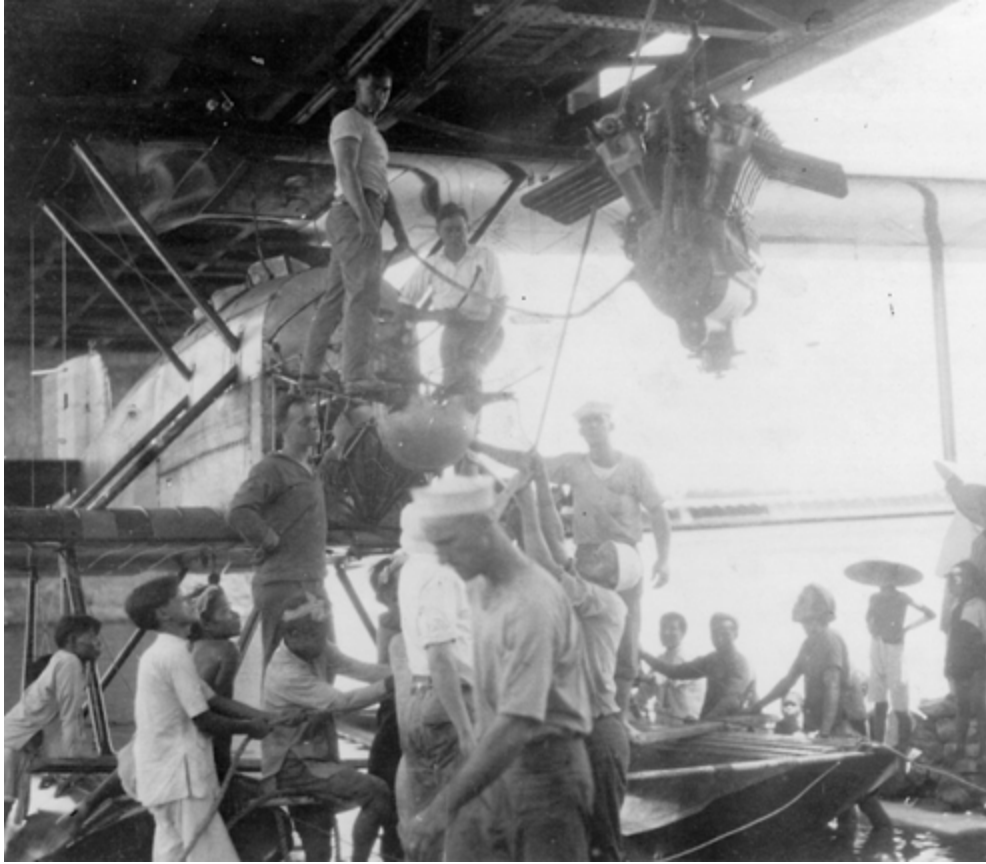
The engine of the Chicago is changed at Hue, French Indochina (now Vietnam), with the help of American sailors under the supervision of Smith and Arnold. The bridge allows for the engine to be dropped into place. (Photo: U.S. Air Force)
