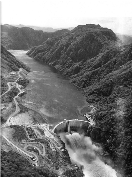
2.3. Cahora Bassa dam in northern Mozambique under construction, December 1976. Picture taken from: Hydroelectric of Cahora Bassa (Eds.). A Nossa Energia Abraça Moçambique – Our power embraces Mozambique: 25º aniversário da hidroelétrica de Cahora Bassa, Lisboa 2000.
