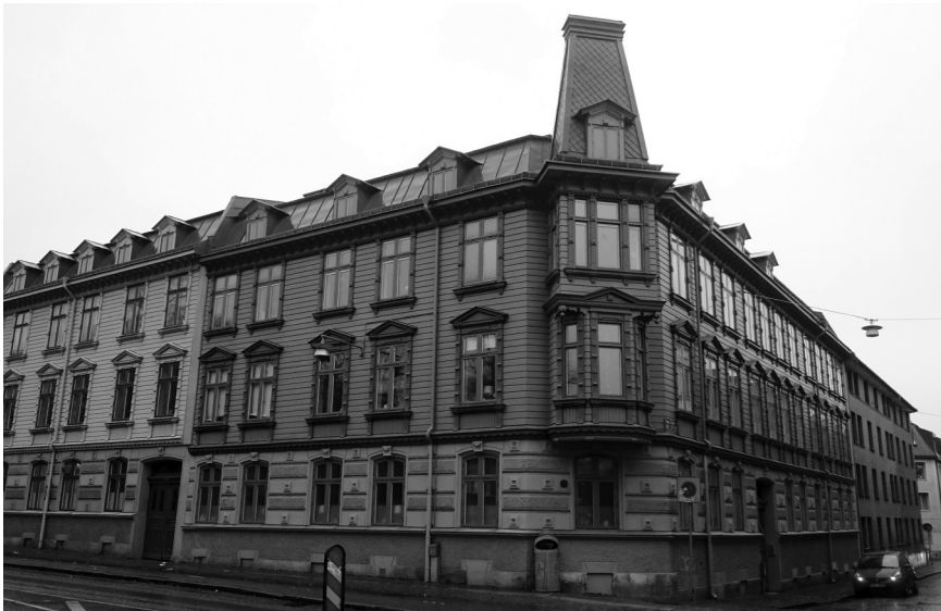
Figure 5.1 The block of Sabeln in Gothenburg, 2017.
