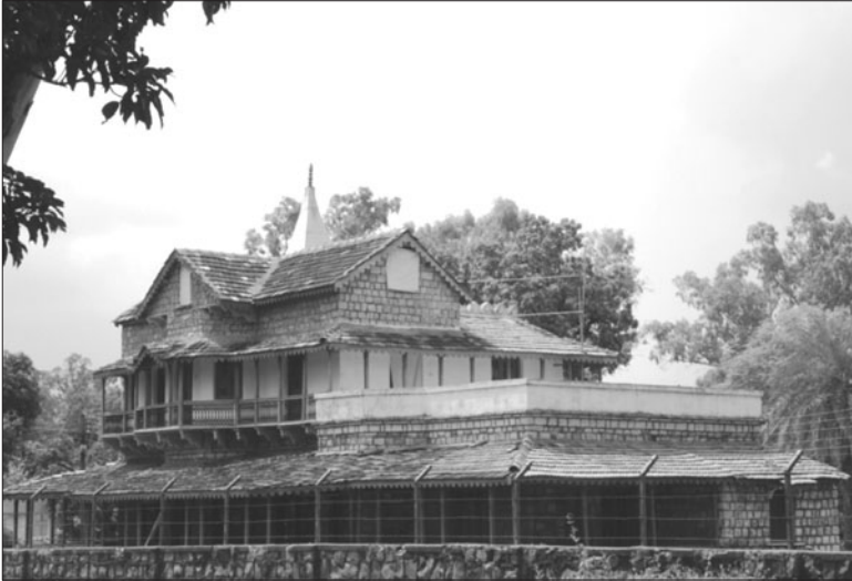
Plate 2.5: John Marshall's house at Sanchi
