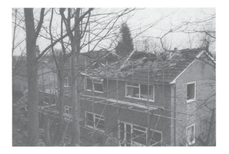
Fig. 16.2. Damage caused by a tree blown over in high winds. Although the roof structure has absorbed most of the impact, there is a need to inspect for any other structural damage. (Jack Hinks.)
