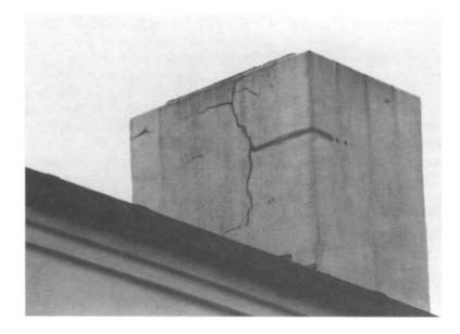
usually only occurs in the external (damp) wall. Internal cracking at weak spots or bowing may occur as the differential expansion of the outer leaf imposes stresses on the inner leaf.
