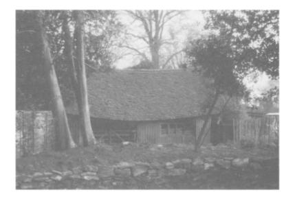
Fig. 13.9. General sagging and distortion of a roof structure. This may be due to overloading or failure of the structure. (K.Bright.)
