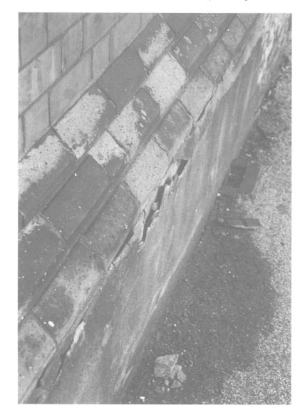
coats are of higher cement content than the undercoats, there exists the possibility of differential shrinkage within the thickness of the multilayered rendering. The stresses generated by such shrinkage may be sufficient to exceed the relatively low tensile failure stress of the render/render interface. Any deficiency in the mechanical keying to the background will increase this possibility. This can lead to the final coat flaking away, sometimes taking with it some of the undercoat.
