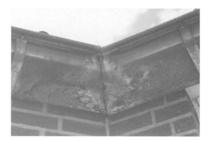
Fig. 5.6. Corrosion of external metalwork. Joints and other stressed regions are particularly vulnerable. (University of Reading.) aluminium. Where water run-off occurs the patina may be washed to redeposit on adjacent surfaces. Clearly, damage by erosion will occur to the patinating metal.
