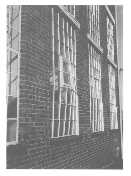
**Fig. 7.3.** Buckling of metal windows due to expansive effect of corrosion.
