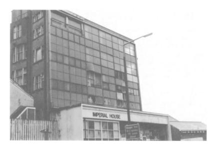
**Fig. 9.26.** Lightweight cladding—intolerance of differential movement between panel and frame. (K.Bright.)
