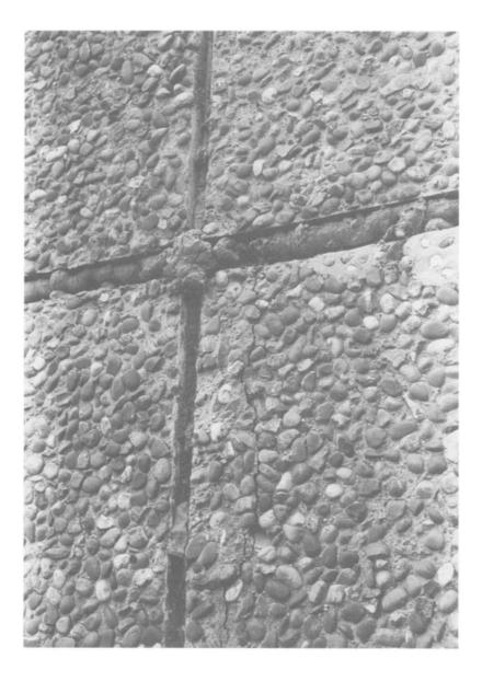
**Fig. 6.6.** The precast concrete panel joints are poorly aligned and of differing widths.
