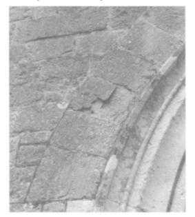
**Fig. 9.13.** Delamination of stone surface. The initial, developing and advanced stages are clearly shown. (K.Bright.)
