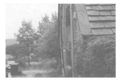
Fig. 10.3. Ballooning of the gable end of a stone building. The downpipe acts as a visual reference line. (University of Reading.)
