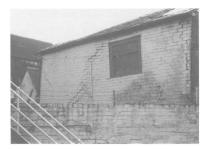
**Fig. 9.32.** Severe diagonal cracking of a solid wall. The external supports appear to be ineffective, although they are evidence of a long-term problem.
