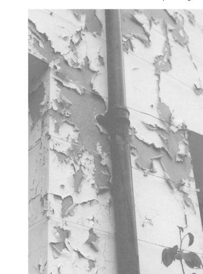
overstress an old, friable base. Particular problems arise between old and new coatings of oil and water-based formulae.
