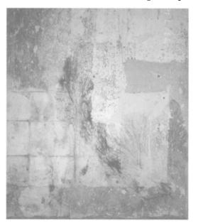
**Fig. 4.4.** General view of the failure, due to dry rot, of a suspended timber ground floor. (S.D.McGlynn.)
