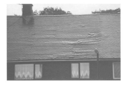
**Fig. 13.12.** General slippage of roof tiles due to nib and nail failure. (D.McGlynn.)
