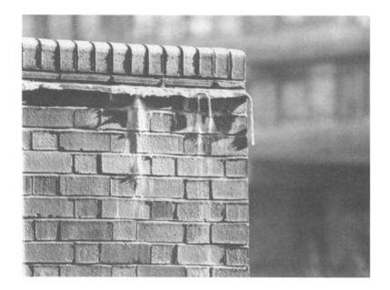
**Fig. 3.2.** The precipitation of soluble salts from brickwork at a DPC may even produce stalactite features.
