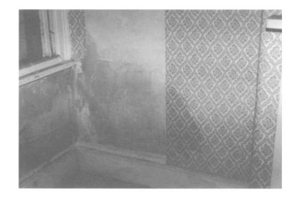
Fig. 9.2. Symptoms of dampness within a building. The general shape and height of the staining suggests that this may be due to rising dampness. (K.Bright.)
