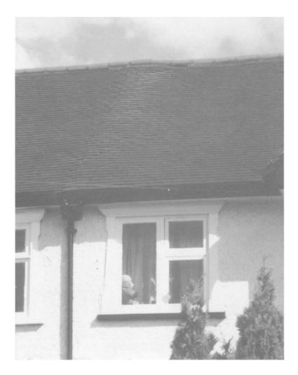
Fig. 13.10. Distortion of roof coverings over a party wall caused by differential movement of the main roof areas. (K.Bright).
