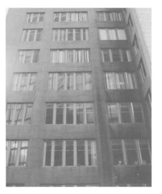
**Fig. 9.16.** The staining of this external façade is more pronounced in the internal corner, where the effect of rain washing is less marked.
