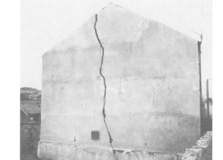
Fig. 8.10. Severe gable end cracking. The crack width increases with height indicating a movement of the lower left-hand corner of the wall.
