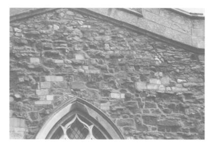
Fig. 9.15. General weathering of stone wall. The pattern of attack has been influenced by the position of replacement stone. (K.Bright.)
