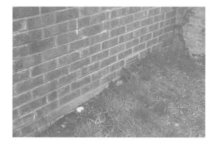
**Fig. 9.8.** The partially buried air brick suggests that the DPC is also close to ground level. (K.Bright.)
