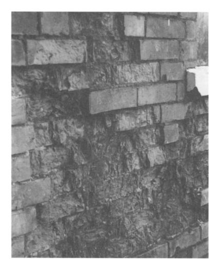
Frost attack in brickwork is usually progressive, causing delamination as the bricks become friable and fail in tension under the build-up of stresses. There appears to be little quantifiable link between compressive strength and frost resistance, except in extreme instances, since the frost attack operates through tensile stresses.
