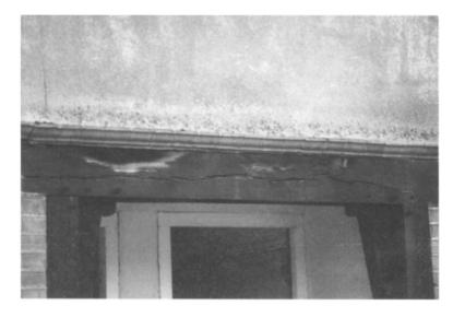
**Fig. 4.1.** External structural timber cracking along the grain. (University of Reading.)
