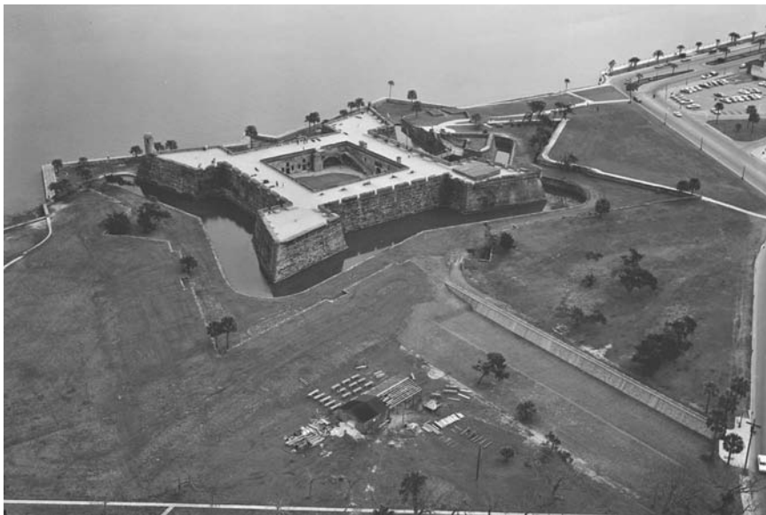
Castillo de San Marcos, Saint Augustine, Florida. Following English and native attacks on Spain's vulnerable outpost this extensive stone fortification replaced an earlier wooden structure. Construction continued from 1672 to 1756. (Library of Congress.)
